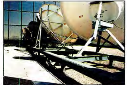
Using a roof-mounted grid allows broadcasters flexibility to update and change outdoor equipment without having to risk damaging the roof membrane.
